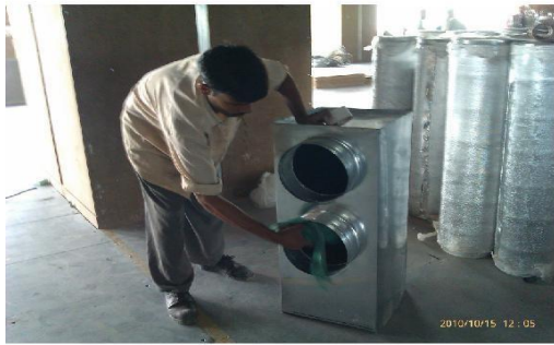
Cleaning Prior To Installation
